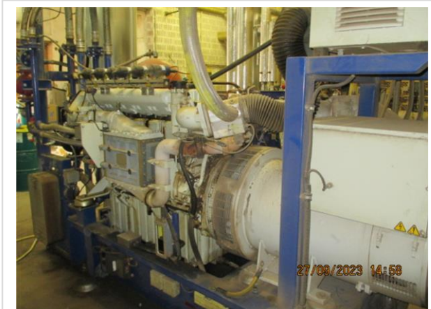
BHKW 2, enertec, 190 kW el.
